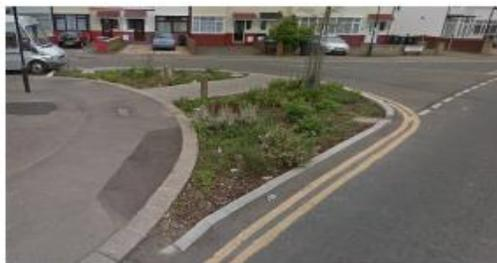
Rain gardens are fed by rain water running off adjacent roads and pavements. By soaking up water and releasing it slowly, they help our sewer system cope better in storm events, minimising flood risk in vulnerable parts of the borough.
